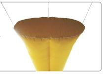
3.Returnsox® use quadruple cable suspension system and Durkeesox® exclusive & patented NIR supporting technology to maintain the flexible air duct in rectangle shape and return air under negative pressure.
